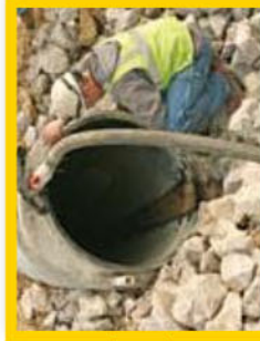
The grout is pumped into the entire length of the pipe, filling in all voids between the new and host pipe, and the areas between the pipe and roadway.
